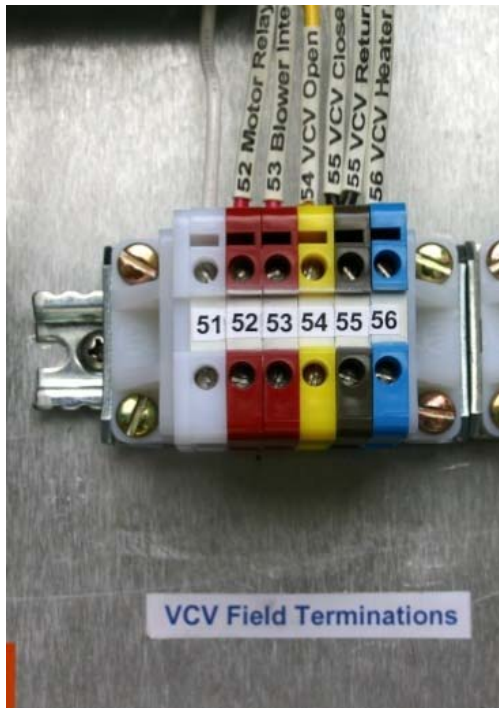
Figure 4 – FALCO Control Box Terminations
